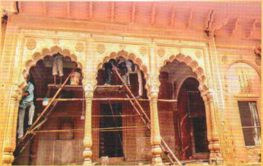
VARDHAMAN KUNJ GETTING ITS FINAL TOUCHES IN REPAIR AND RESTORTION
