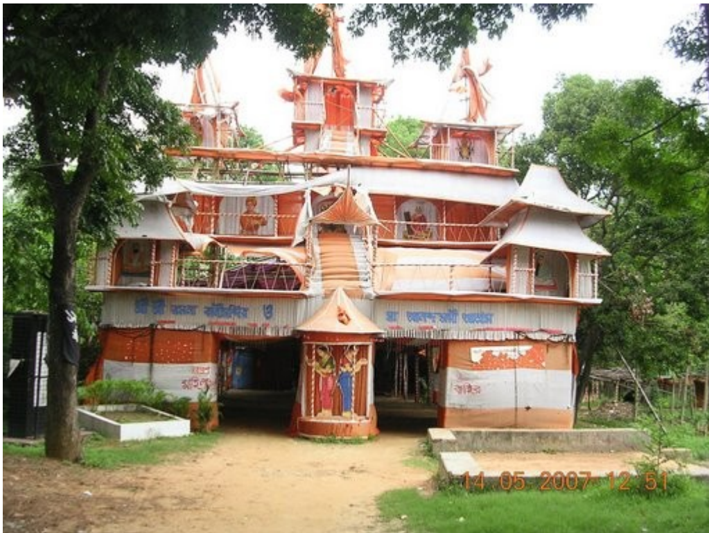
Temporary pandal erected on part of the original Kali temple/Ramna ashram site
